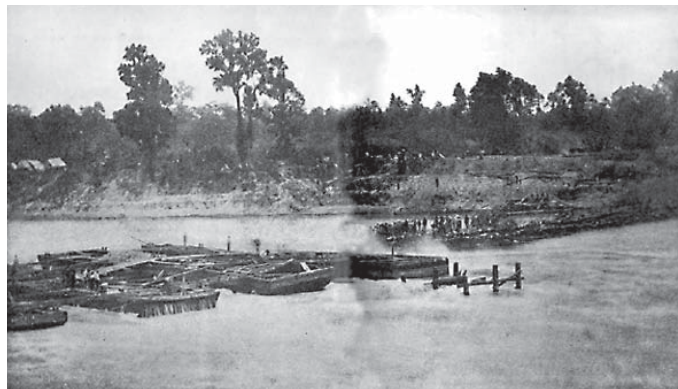
Bailey's Dam under construction, May 1864
